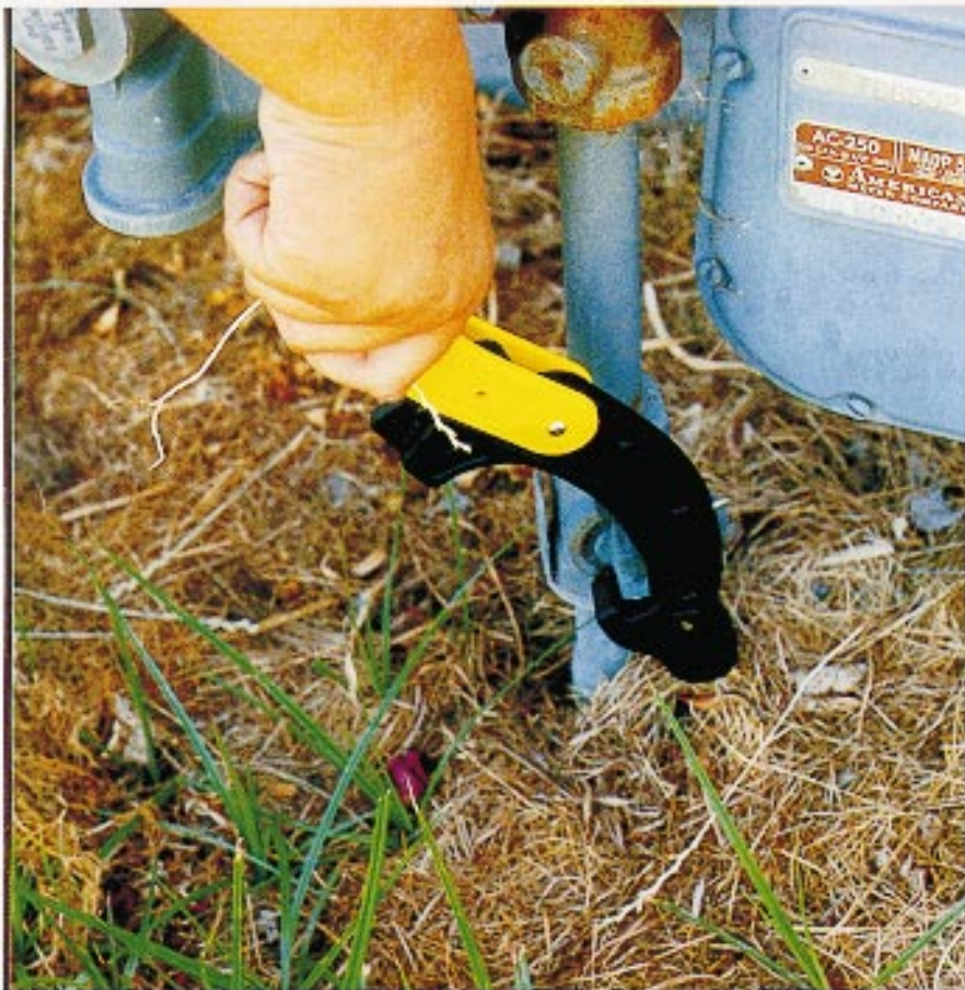
The spanner can shut off a gas line.
