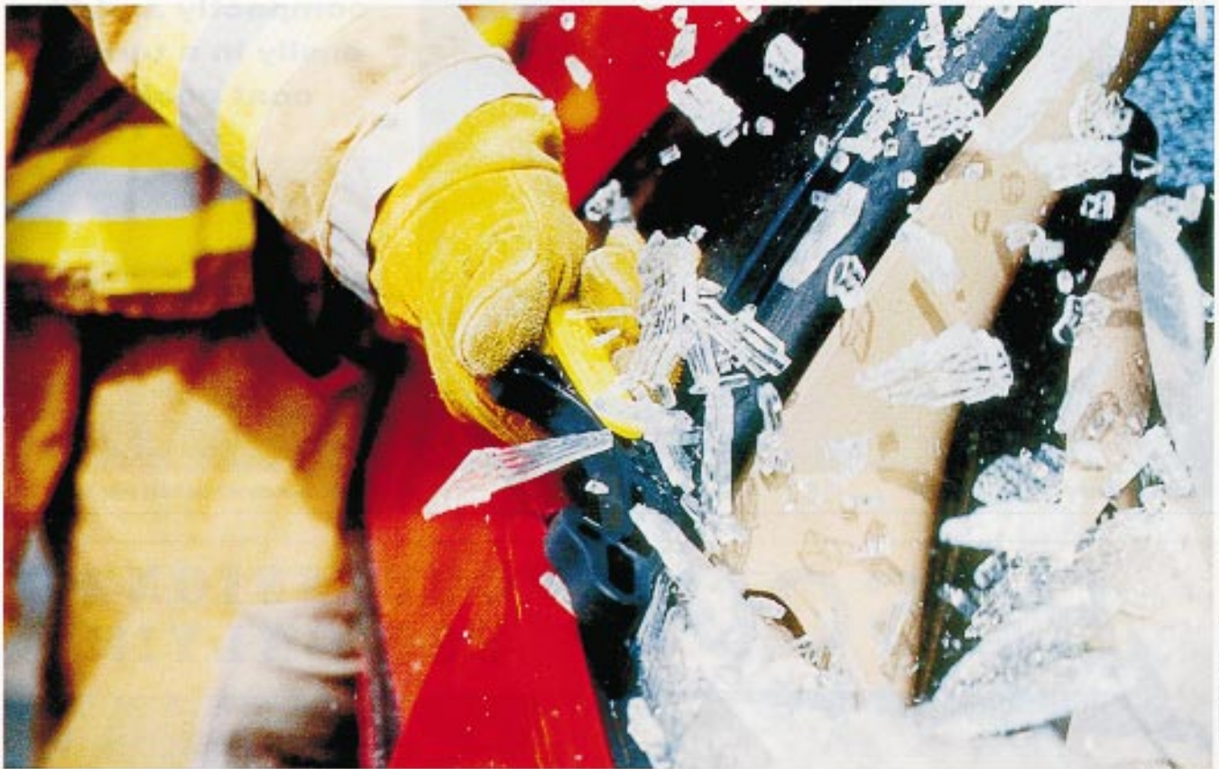
Rescuers can bust out a tempered glass window with Res-Q-Rench.
